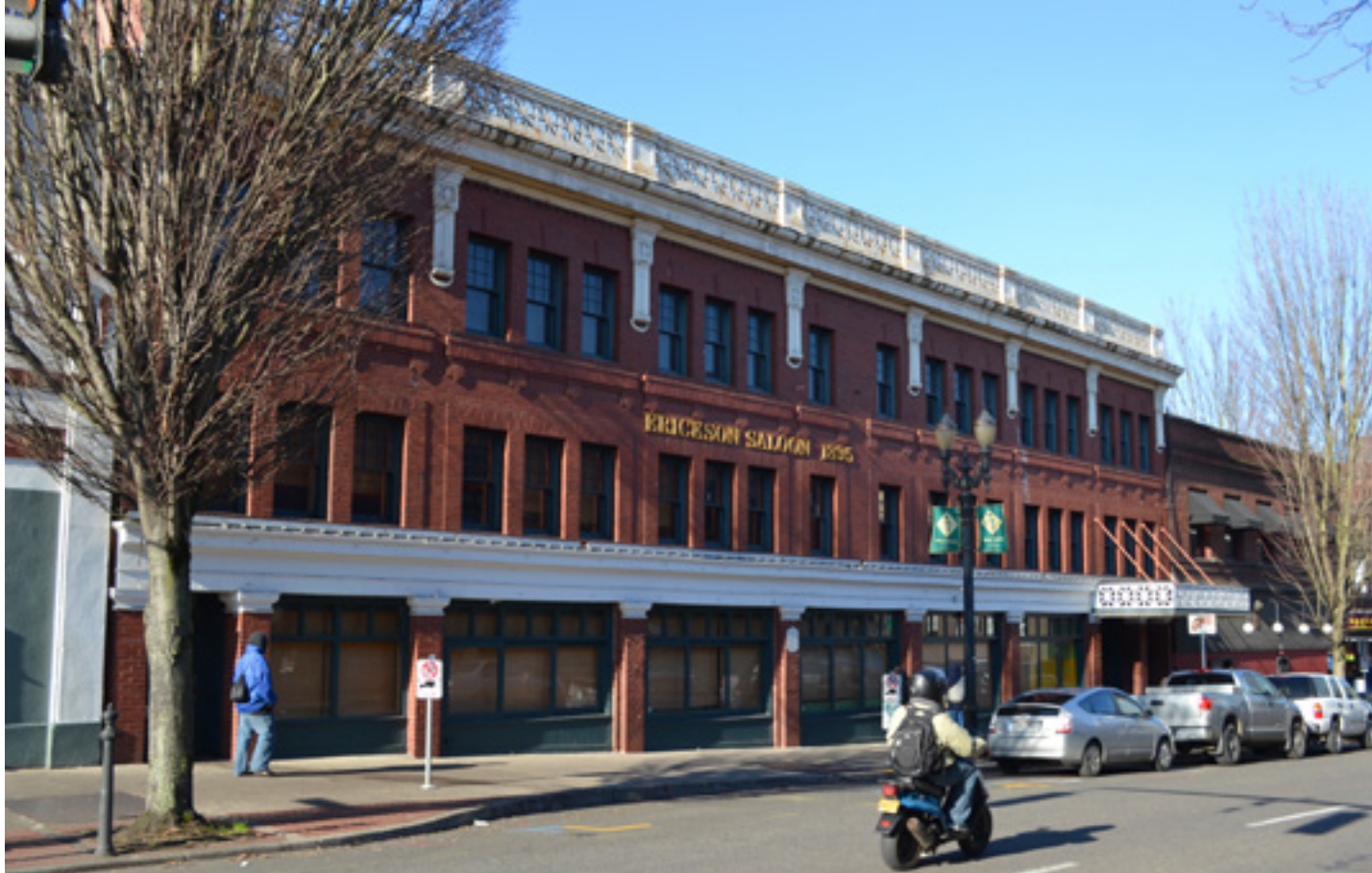
The storied Erickson's Saloon building is about to get a new use—housing. Photo by Donald R. Nelson
